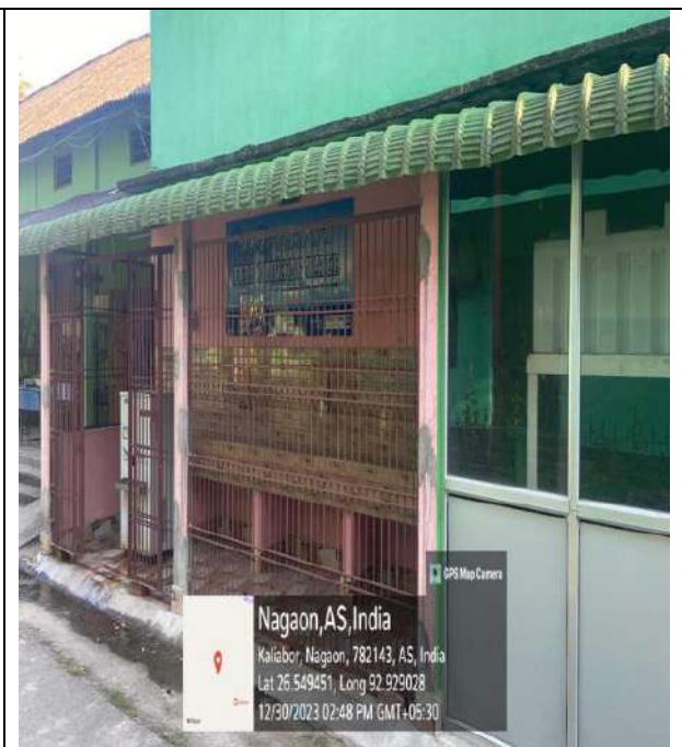
The Drinking water Plant
