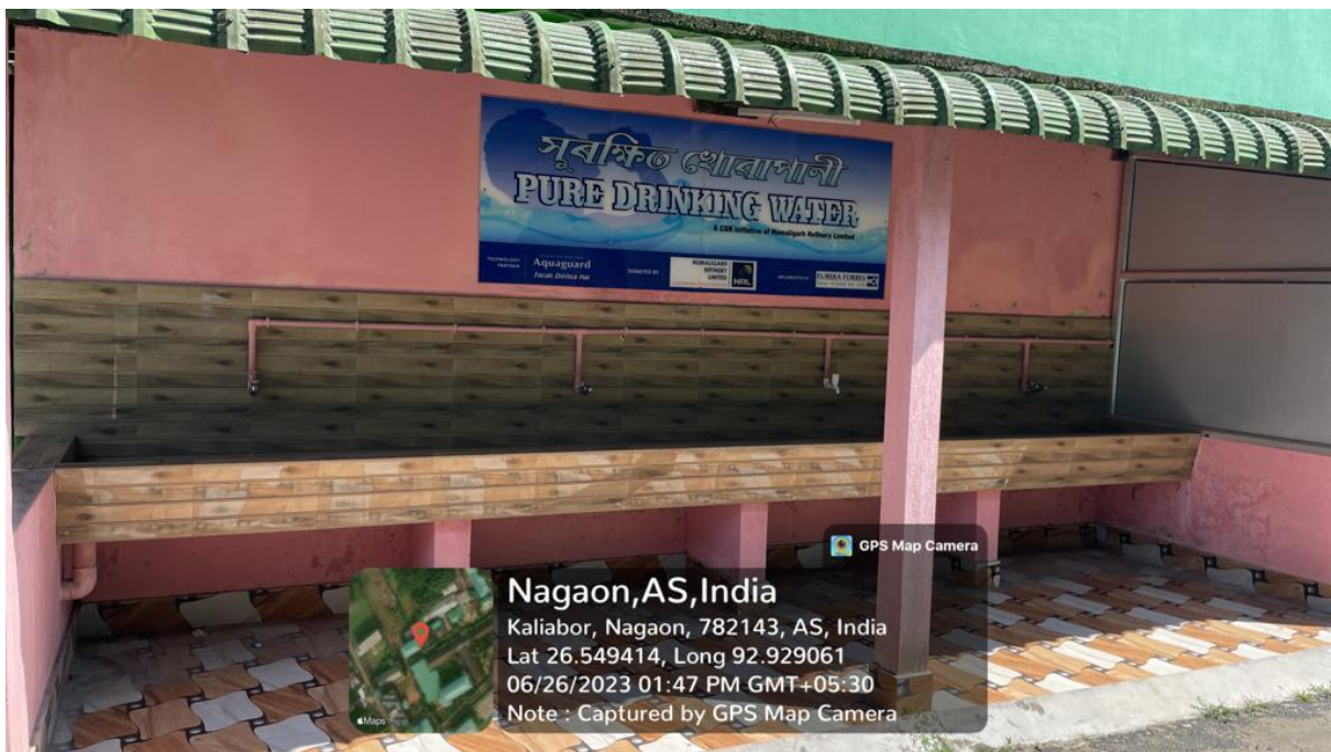
DRINKING WATER FACILITY
